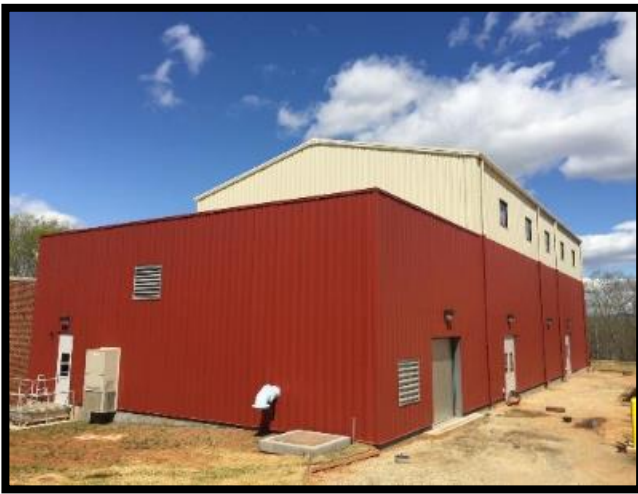
South Rivanna WTP
