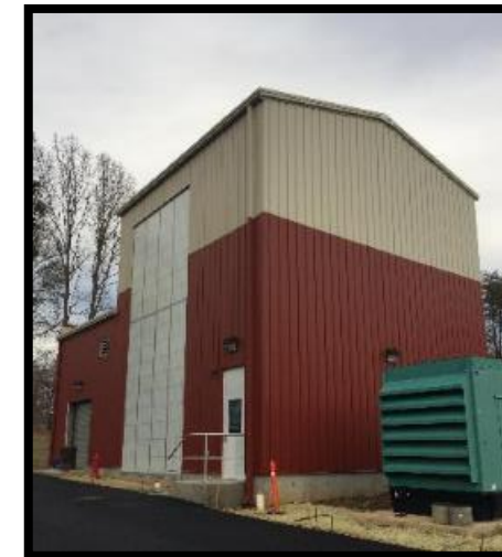
North Rivanna WTP
