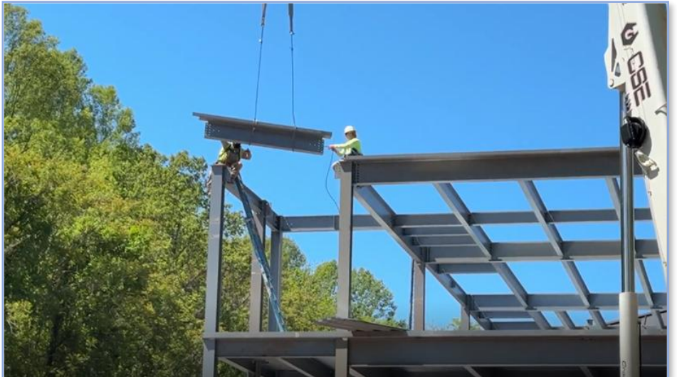
Installation of the beam on the top of the building addition
