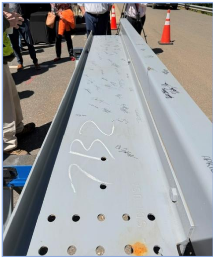
Final Steel Beam with Signatures of Attendees
