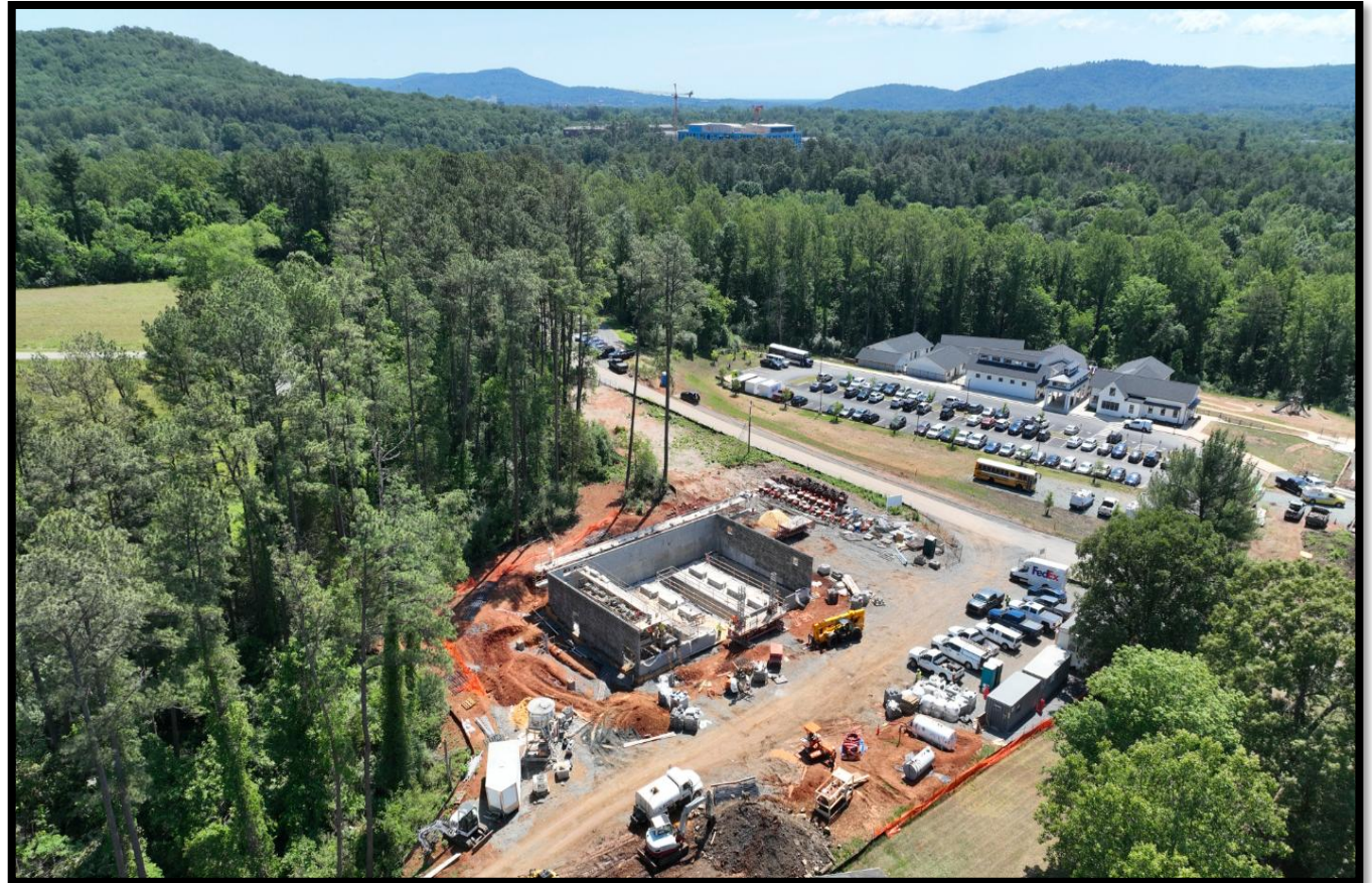
Ragged Mountain PS Construction on Reservoir Road
