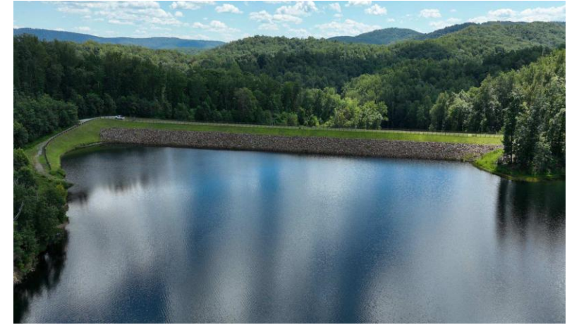
Ragged Mountain Reservoir and Dam
