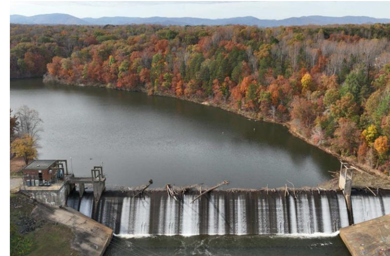
South Rivanna Reservoir and Dam
